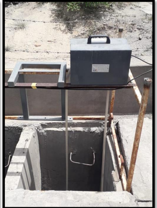
Fig 06- State of the art ETP in working condition with Oil Skimmer
