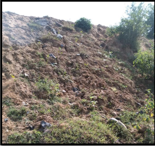
Fig 04- Plantation and grassing along the slopes of the Embankment
