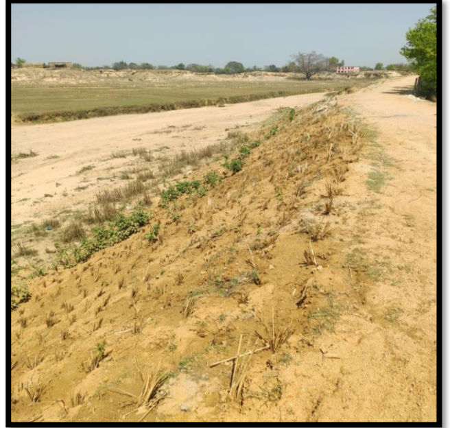
Fig 04- Plantation and grassing along the slopes of the Embankment
