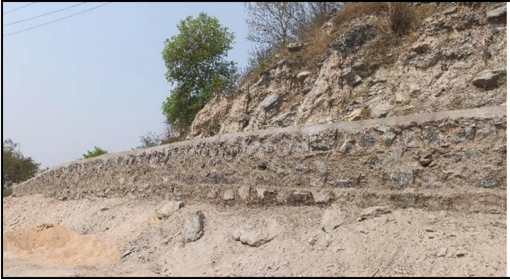
Fig 10 – Newly constructed Toe Wall along the Dump
