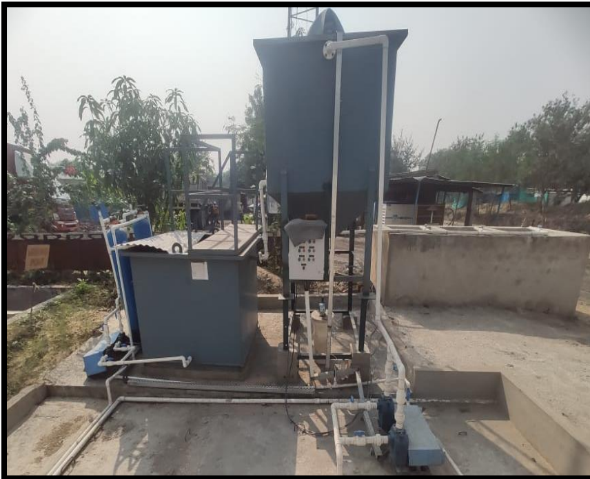
Fig 06- State of the art ETP in working condition with Oil Skimmer
